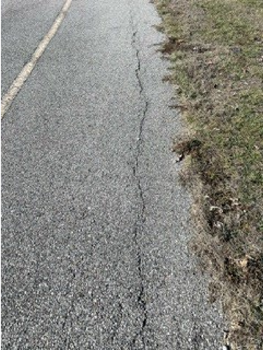
LONGITUDINAL CRACKING EXAMPLE
