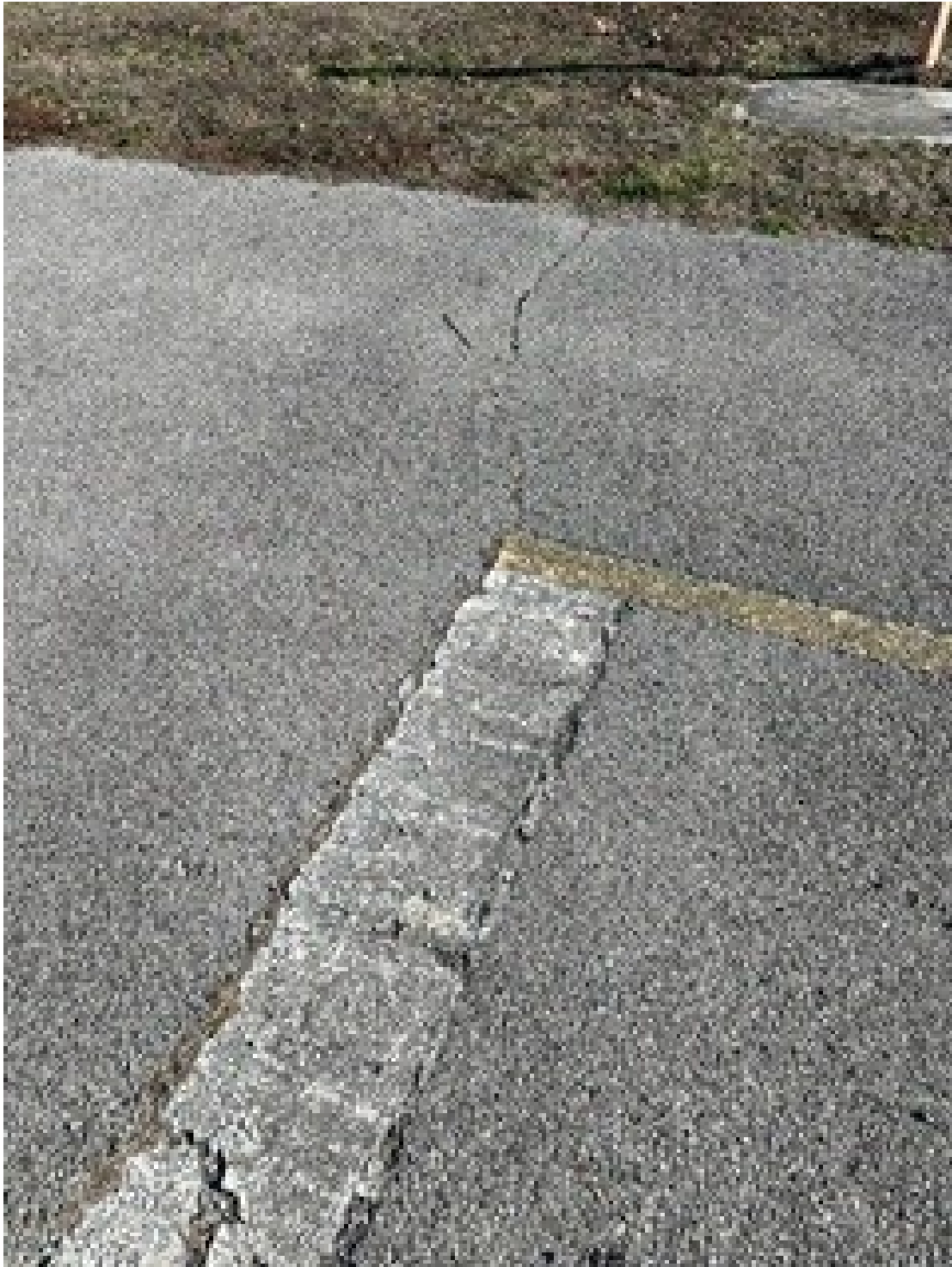
TRANSVERSE CRACKING EXAMPLE
